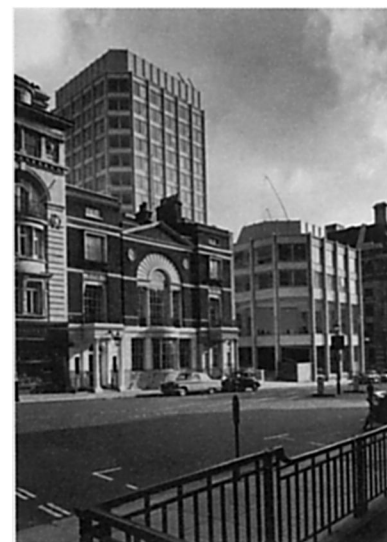
9. Economist Building: View down St James's Street.
